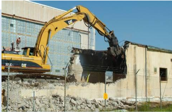
4,500 facilities to decontaminate and demolish
