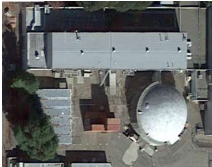
LLNL– Livermore Pool Type Reactor Building 280
