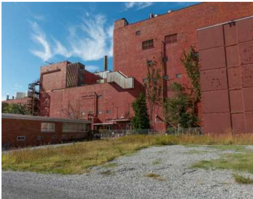
Y-12 National Security Complex – Biology Complex Building
