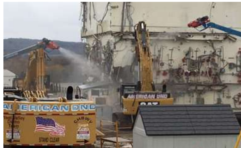
Demolition of WVDP Vitrification Facility
