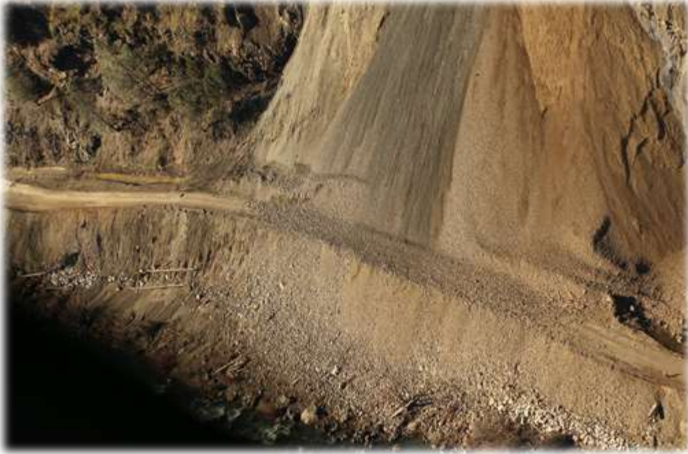
2017 Highway 299 Landslide Credit: CalTrans
