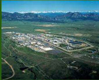
Rocky Flats Before
