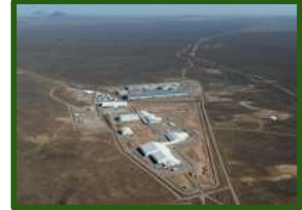
AMWTP at Idaho
