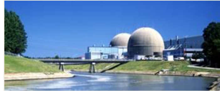
Surry Power Station
