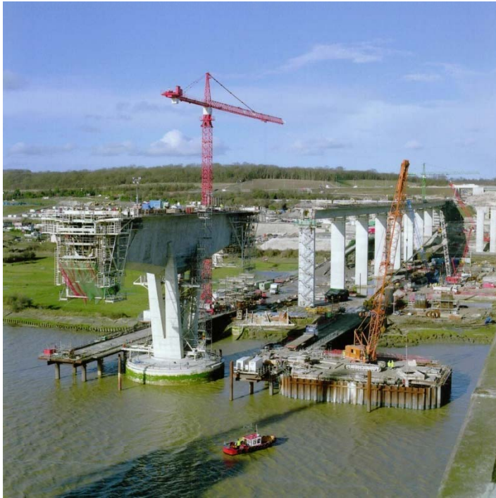
1.2 Km Medway Viaduct under construction
