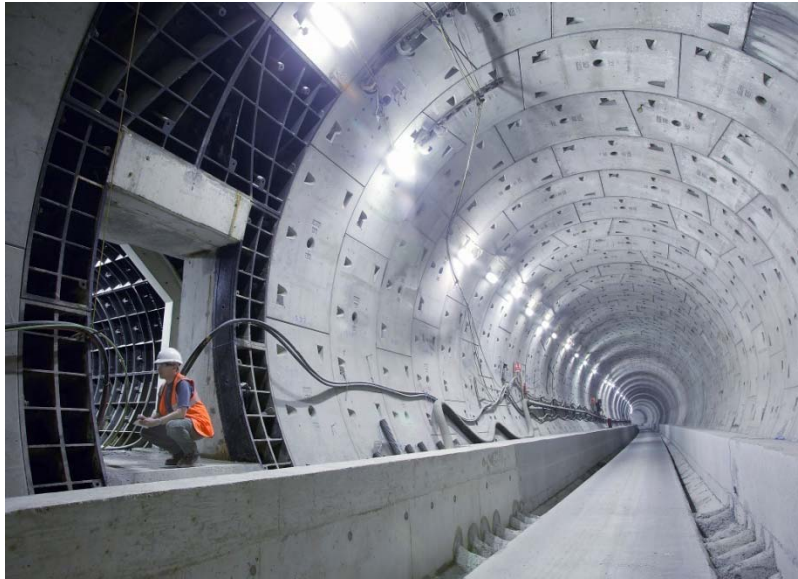
Completed Thames tunnel ready for track laying
